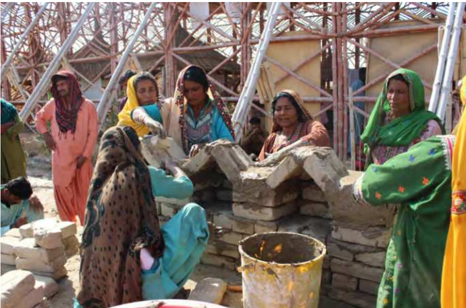
WOMEN LEARNING CONSTRUCTION TECHNIQUES AND MAKING MUD BRICKS © HERITAGE FOUNDATION OF PAKISTAN
