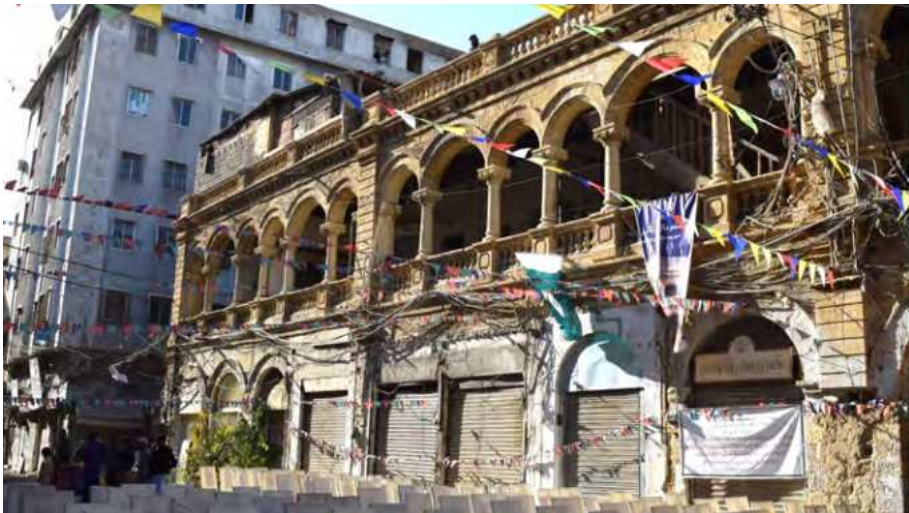
REGENERATION OF HISTORIC CORE, DENSO HALL RAHGUZAR WALKING STREET, KARACHI, PAKISTAN, 2019-2021 © HERITAGE FOUNDATION OF PAKISTAN
