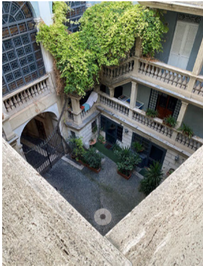
Figure 1 The office courtyard
